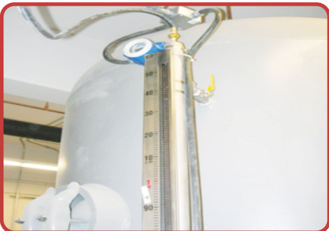
Level gauge coupled with an Magnetostrictive level transmitter
